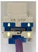
Push the two parts firmly together & trim off excess wire ends.
